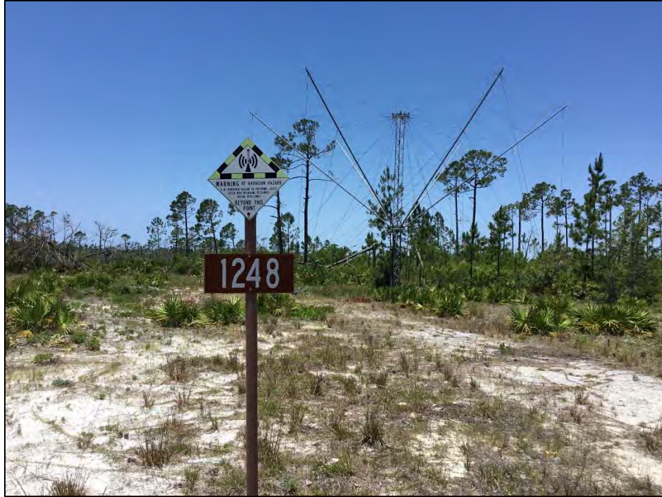
Figure 6. Antenna with radiation hazard sign, facing southeast.
