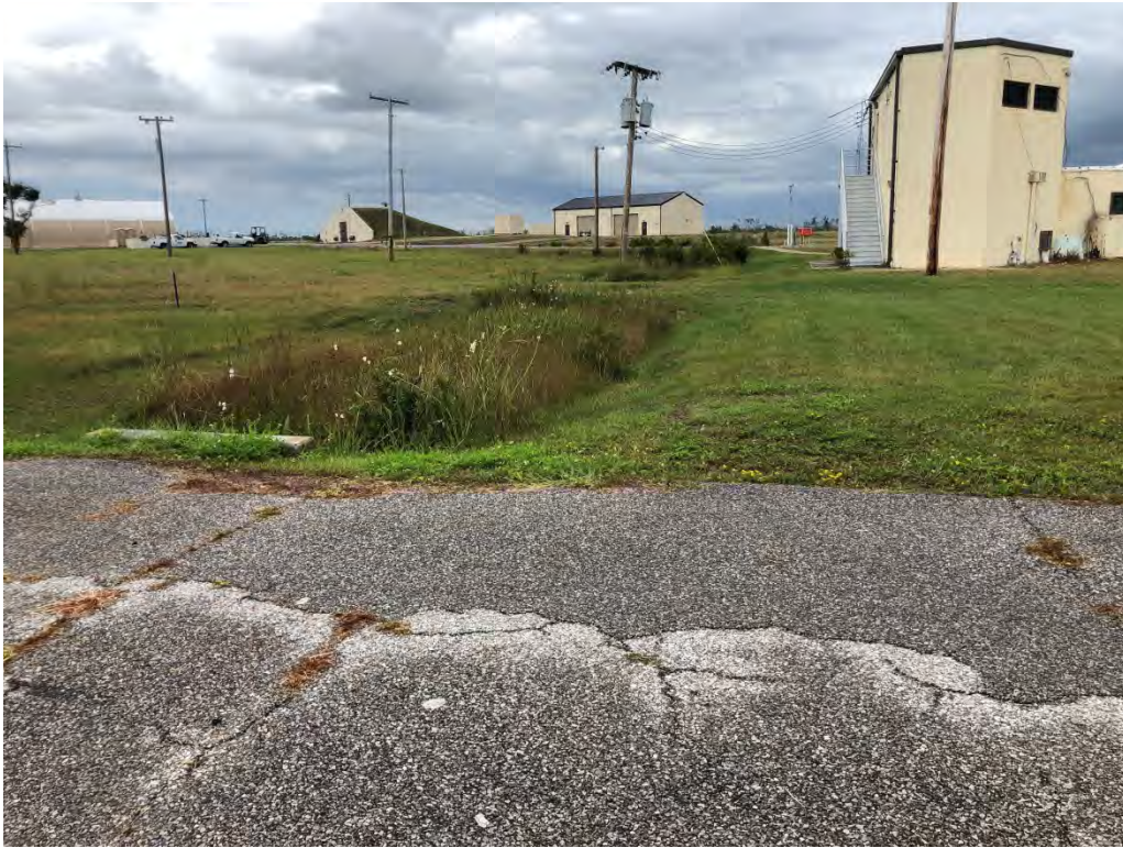
Photograph 9. 8500 Area showing buildings, bunker, and paved road facing north.
