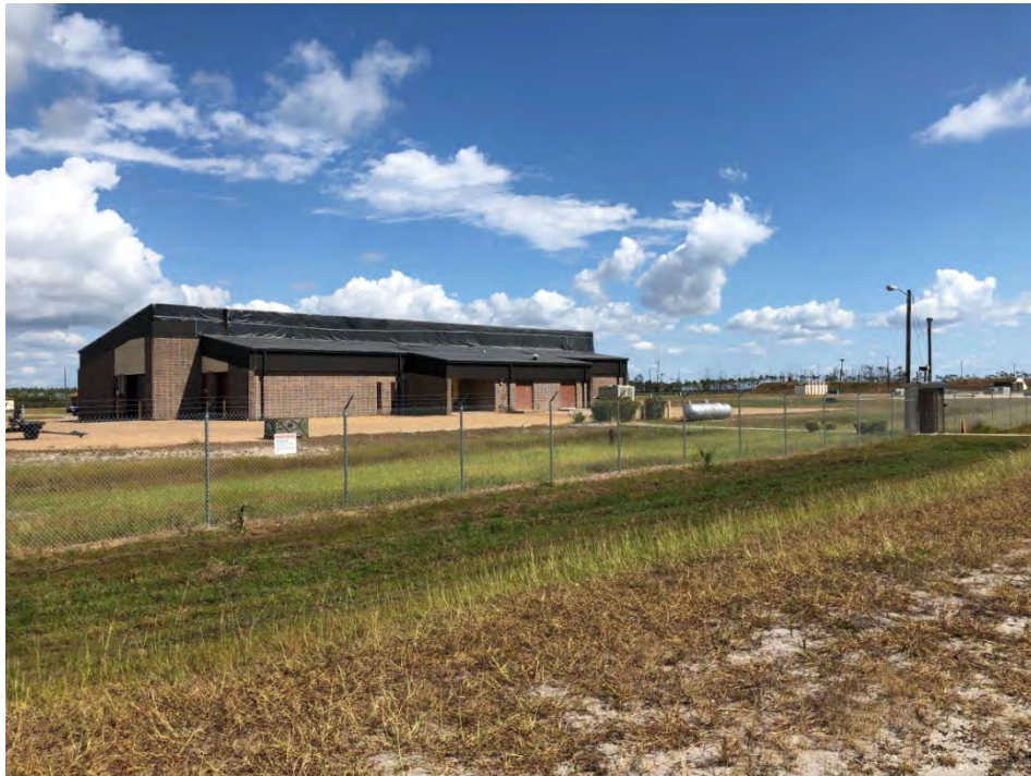
Photograph 7. Munitions building inside perimeter fencing with earthen bunkers in background right view from unnamed road facing north.
